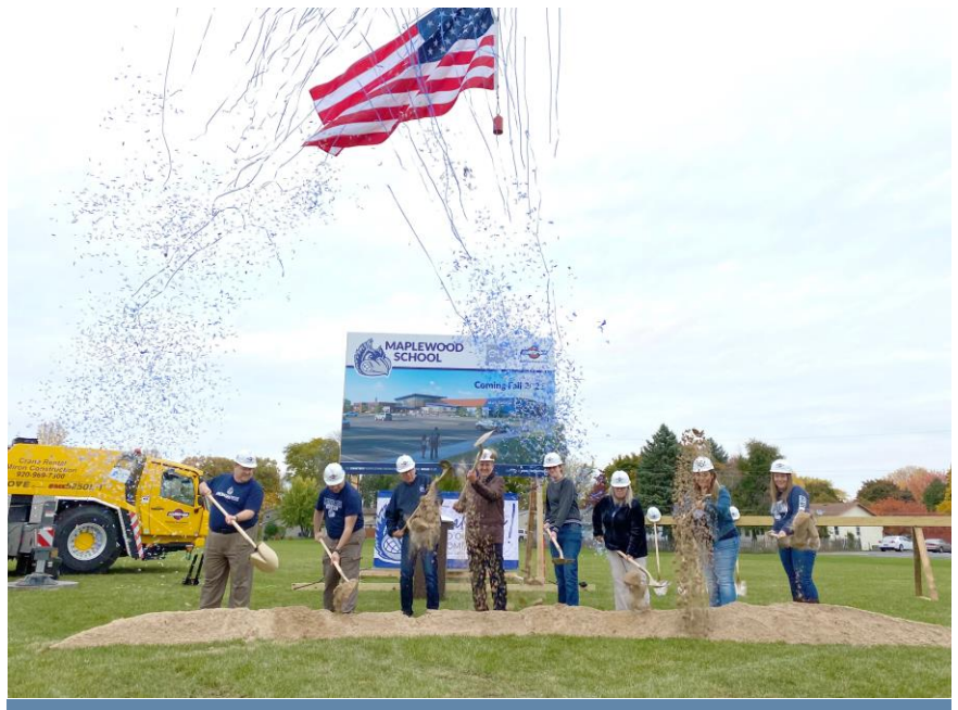
Menasha Joint School District Board of Education members lead the ceremonial shovel turn at Maplewood School.
